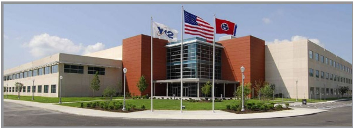
Figure 1. Y-12 National Security Complex New Hope Center
